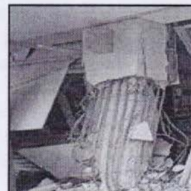
Fig. 2(g): RC Column (Northridge 1994)
